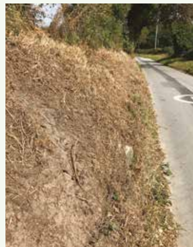
Was it really necessary to remove nearly all of the growth from this banque?
